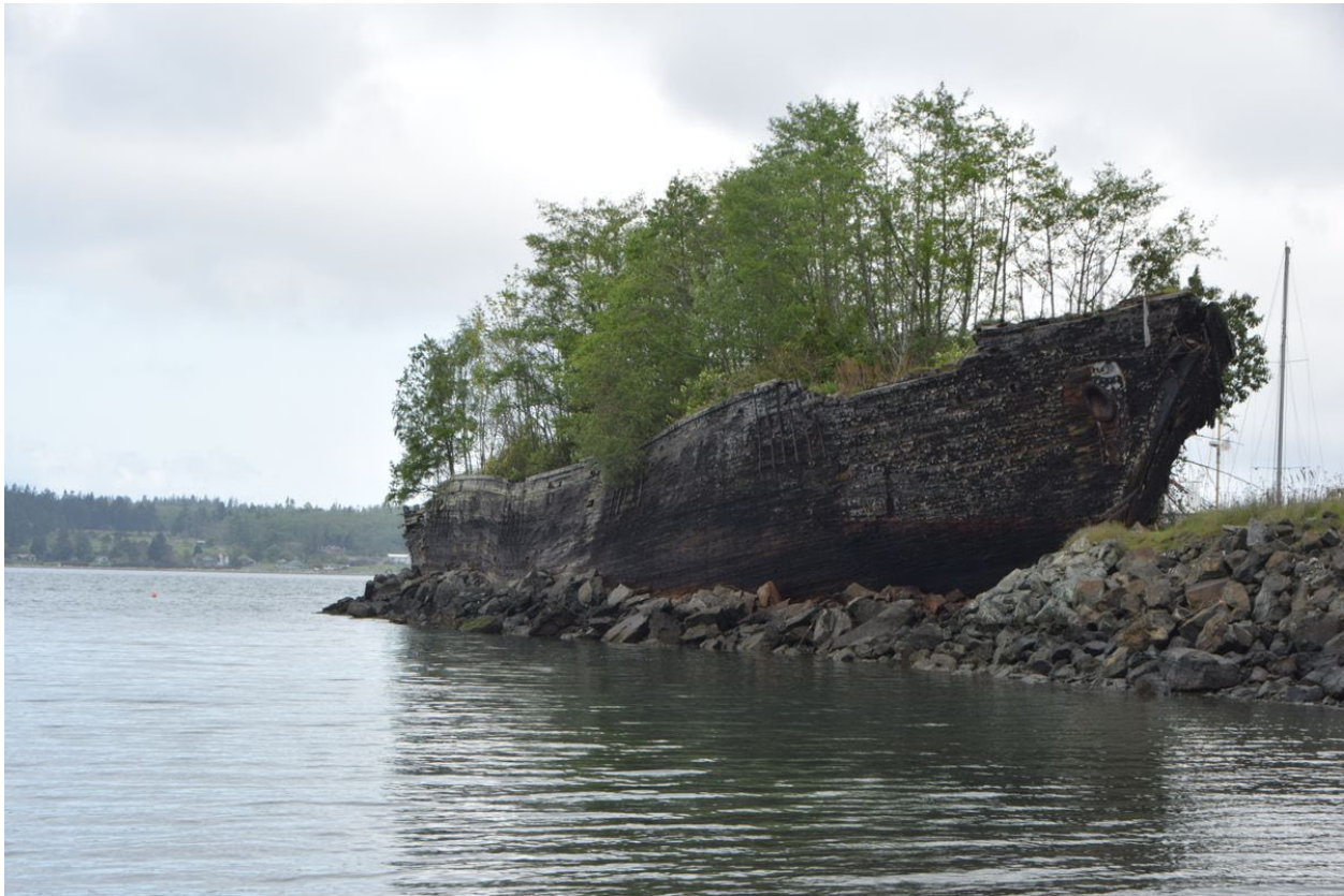
Figure 17. La Merced Historic Vessel used as portion of breakwater
