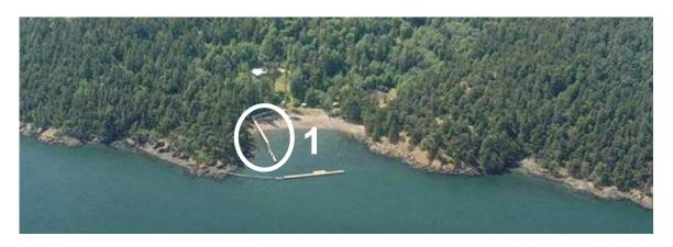
1. 37 Fixed piles in use for dock. Each pile averages about 240" x 12" dia. In addition, about 20 creosote timbers averaging 120" x 12" x 2".
