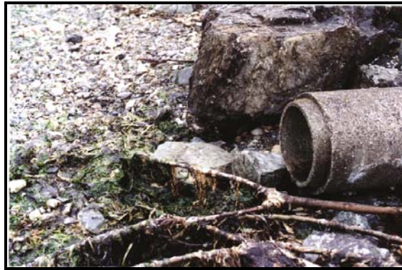
Figure 7: Freshwater discharges entering the nearshore environment can carry excess nutrients or toxic pollutants onto the beach.
