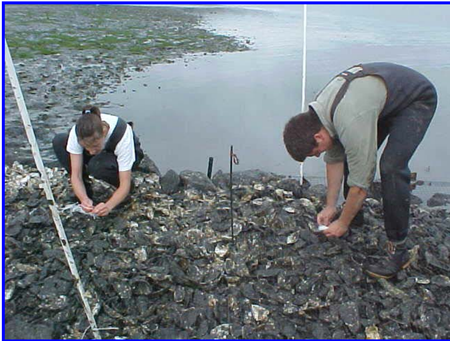
Fig. 3. Laying seeded cultch in the shell mass forming the body of the artificial reef.
